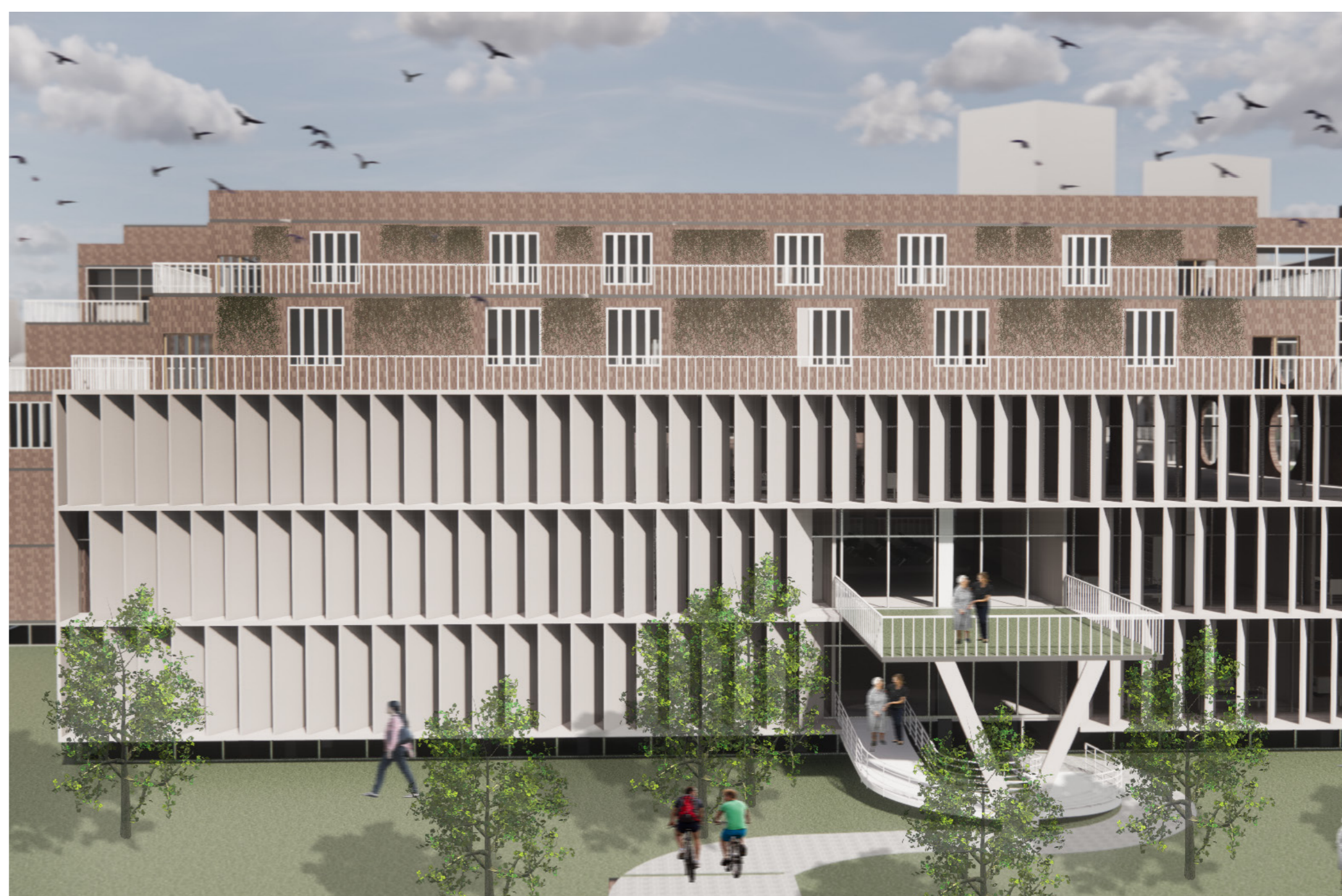
LOUVERS ON FACADE
