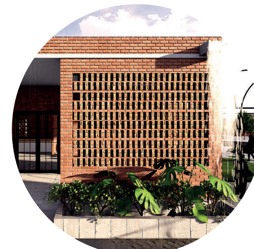
brick jaali wall and a concrete gargoyles pouring rainwater into the planter bed
