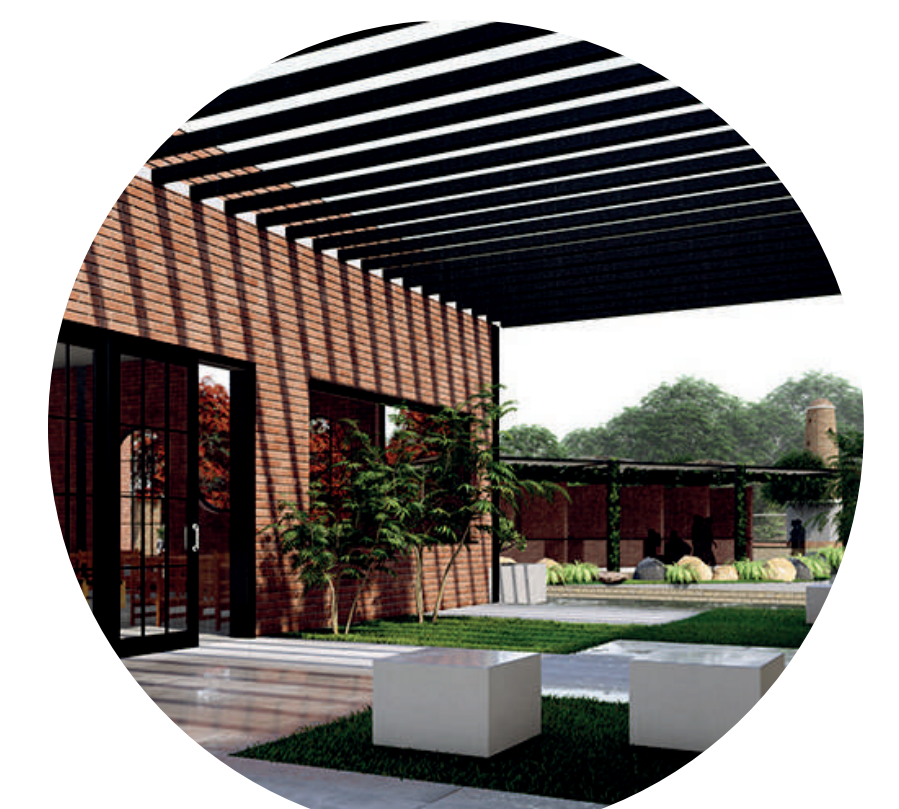
A 6m wide space covered with pergolas between two units act as a spillover
