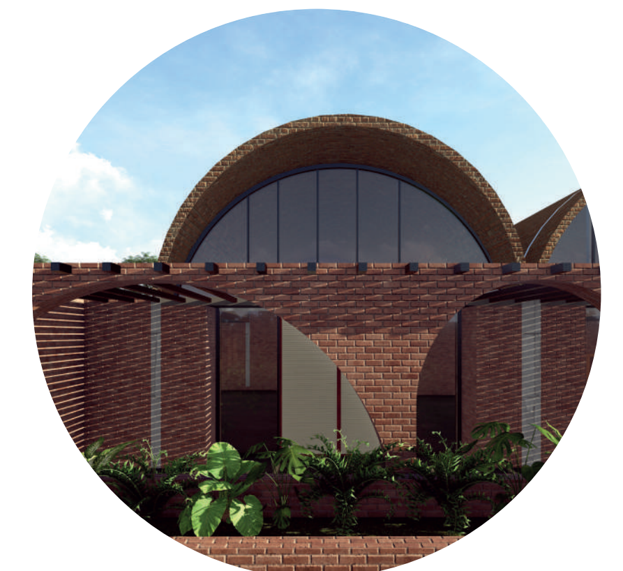
The vaulted roof is projecting outwards to prevent heat gain
